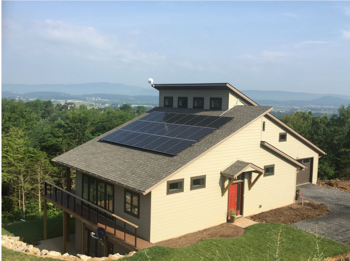
Newly constructed Case Study home, located in Virginia at 38 degrees north latitude. Note 7.2 KW solar PV array on southern roof; there are also passive solar elements on three levels.
